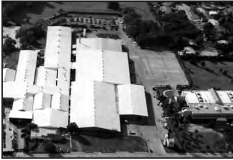
Our Headquarters operation in Arlington, Texas serves as backup inventory for our Service Centers throughout North America.
