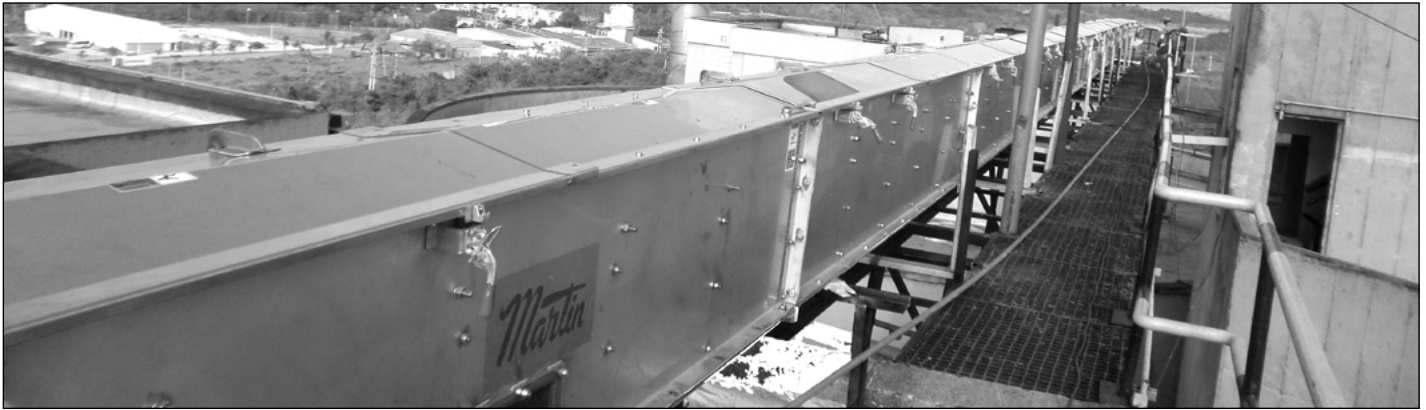
Field assembly of Martin MFB™ Drag
